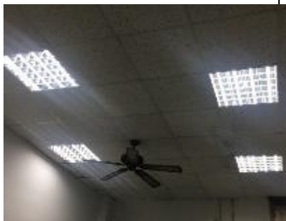
照明系統更新為省電 LED
